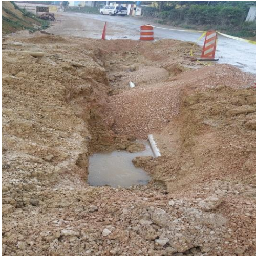
NWC pipe line replacement works in progress
