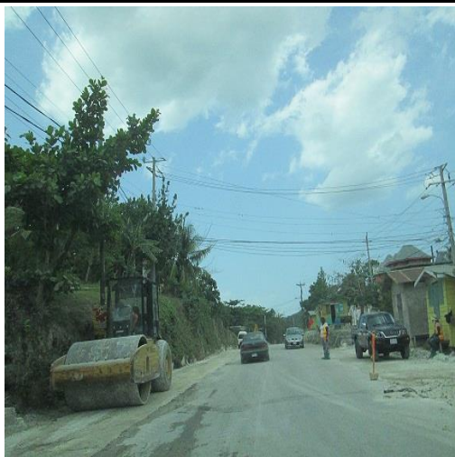
Compaction of Base Course Material to the soft shoulder of a section of the roadway
