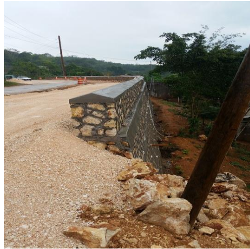
Backfill to recently constructed retaining wall
