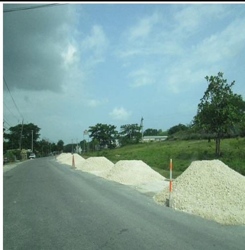
Base Course Material deposited along the soft shoulder of a section of the roadway
