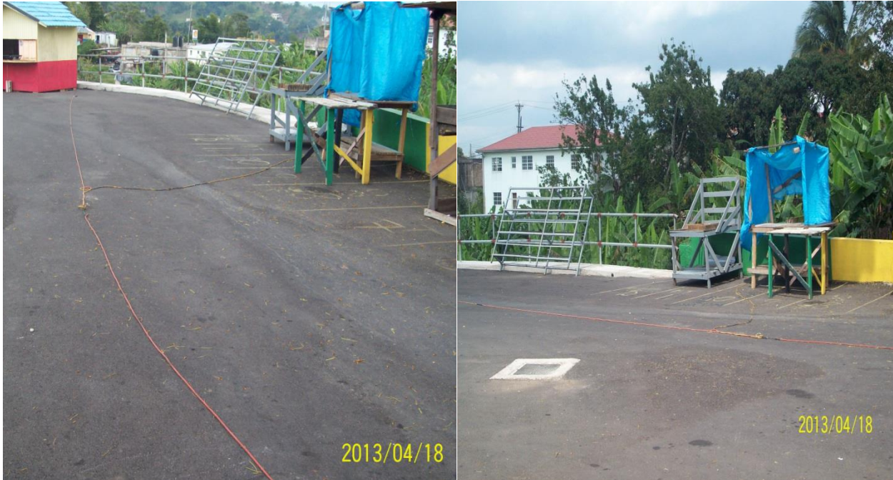
Pictures identifying an electrical connection from the concrete structures located in the sub-basement of the Market providing electricity to certain of the wooden shops
