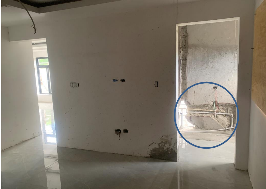
Appendix #5 – En Suite bathroom on ground floor with plumbing works ongoing
