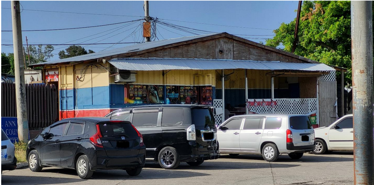
Frontal view of the concerned construction seen from the left.
