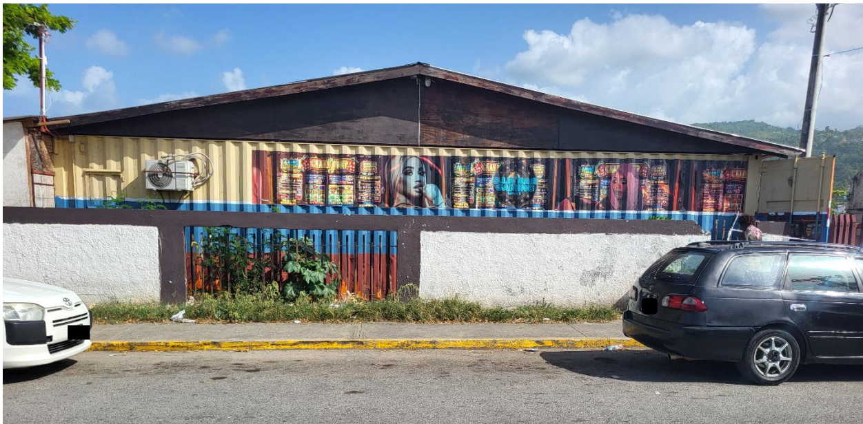
View of the concerned construction seen from the rear.
