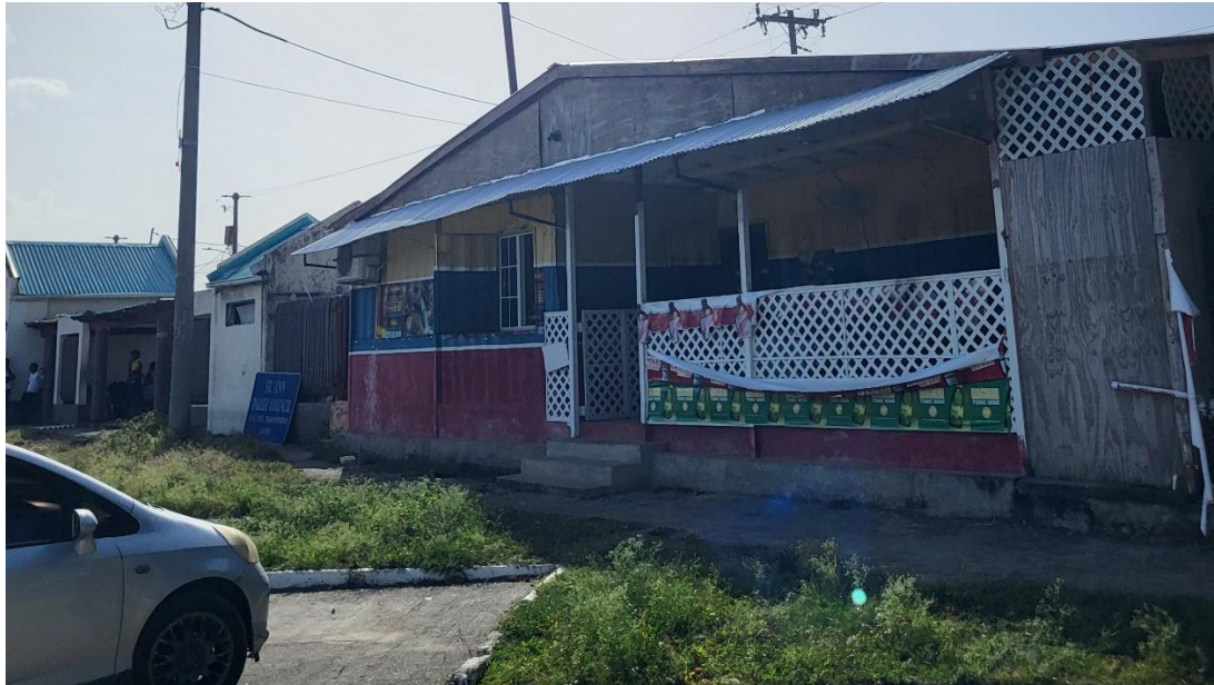
Frontal view of the concerned construction seen from the right.
